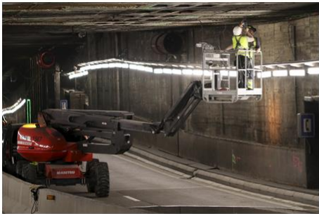
Installation of automated monitoring system in the Rogier tunnel in Brussels
