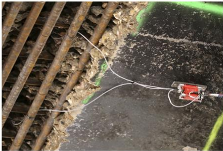
Installation of automated monitoring system in the Rogier tunnel in Brussels
