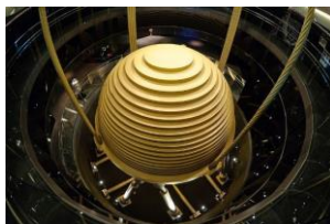
Figure 1. Tuned mass damper at top of Taipei 101 building (taken from https://www.atlasobscura.com/places/tuned-mass-damper-of-taipei-101 )
