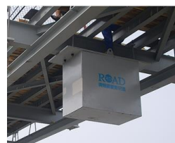
Figure 2. The TMD used in the passenger foot-bridge (taken from http://www.roadjz.com/en/show.asp?id=18 )
