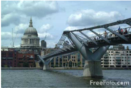
Millenium Bridge (London)
