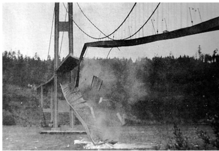
Collapse of the Tacoma Narrows bridge
